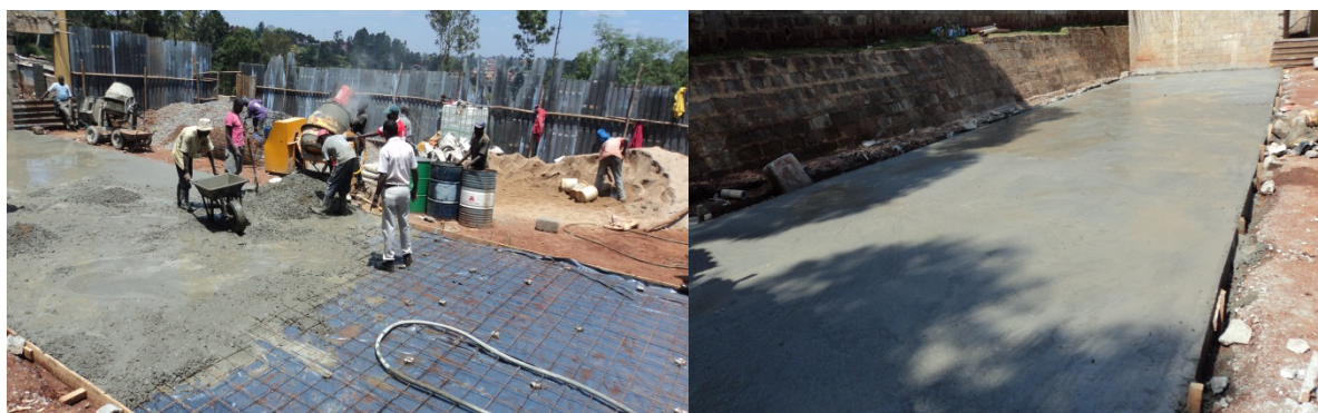
Doing the ground floor slab
