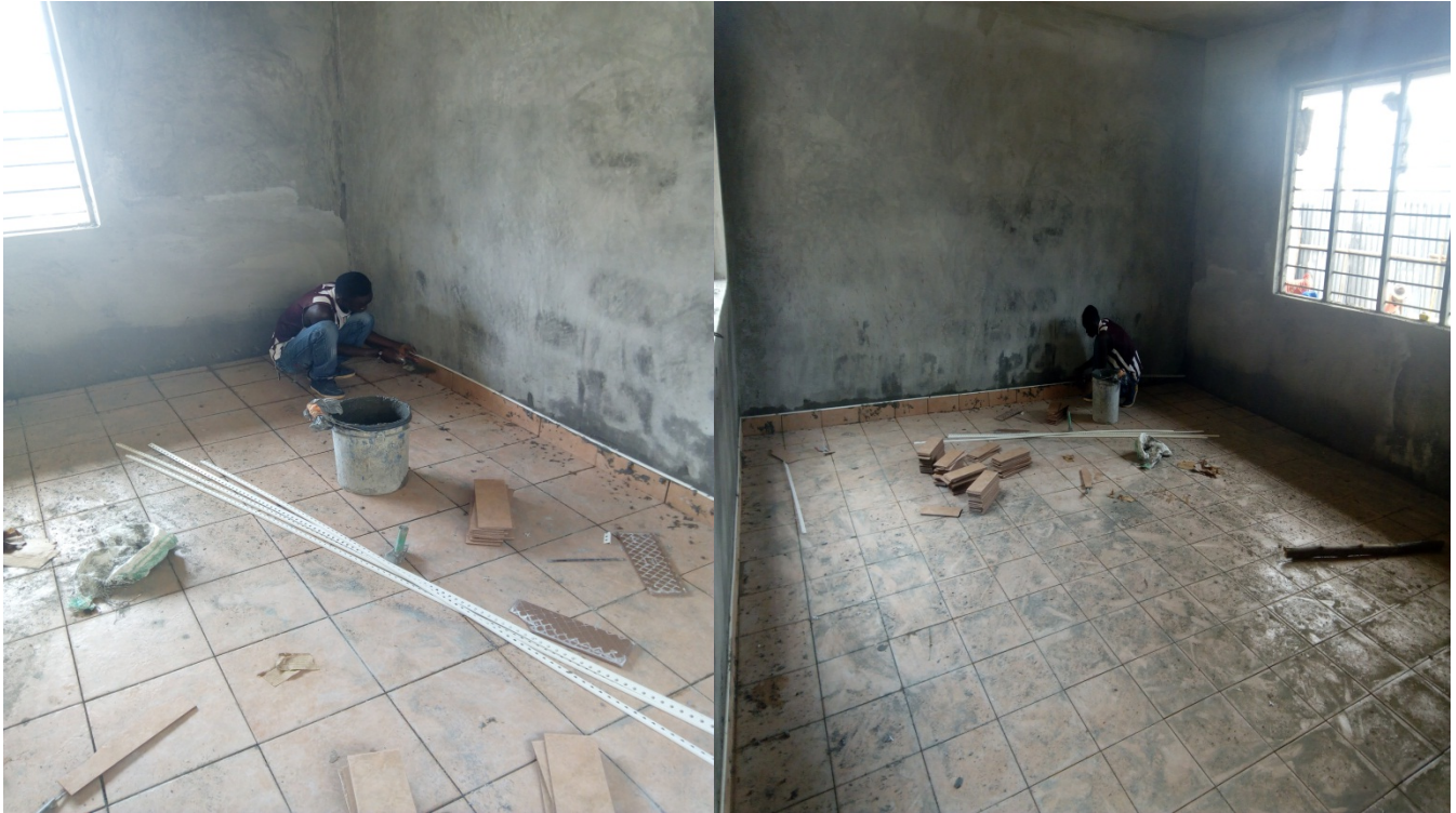
Fixing of the tiles
